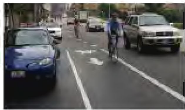
BIKE LANE Establishes space on road exclusively for bicycle travel. Bicycle lanes are striped and marked with a bicycle symbol and an arrow. PHOTO: Active Transportation Alliance
