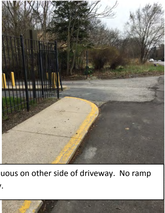
Driveways are not flush and present discontinuity issues
