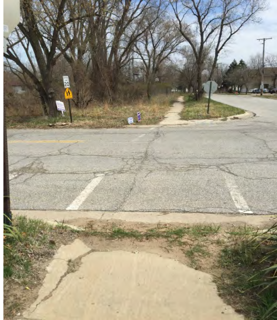
Crosswalks markings faded or missing
