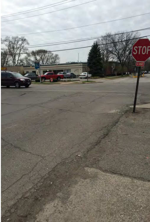
Crosswalks markings faded or missing
