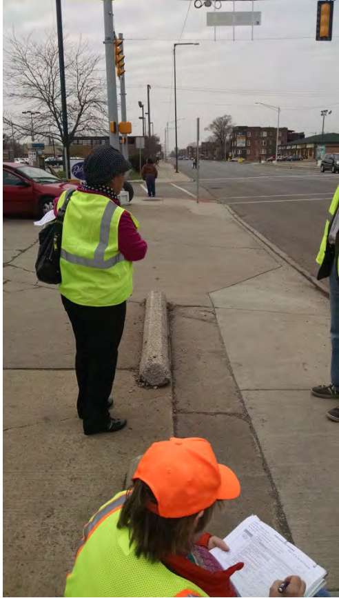
Gas station's driveway has encroached on sidewalk
