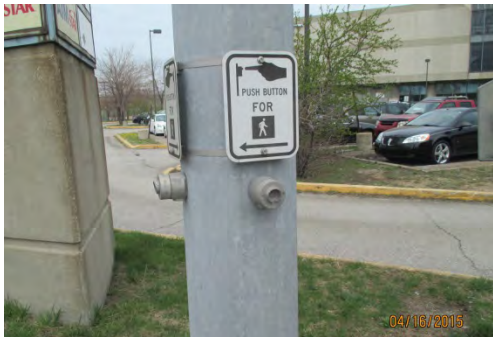
Pedestrian push buttons are recessed not domed along route. Road was reconstructed in 2012.
