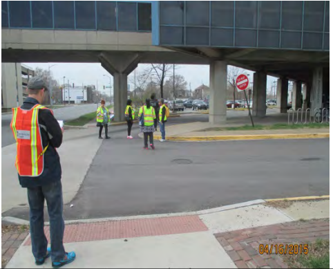
At Gary Metro/ NICTD Station there are no crosswalks or ramps to entrance
