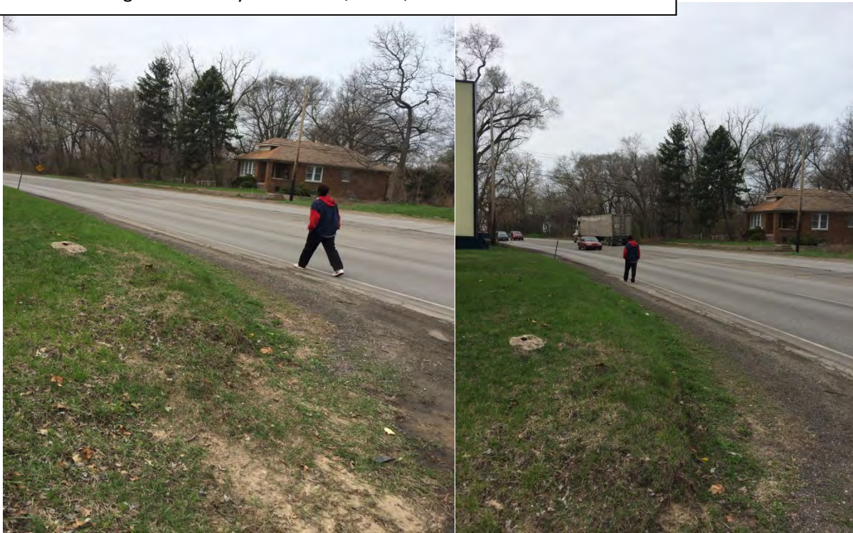
No sidewalk present but pedestrians & bicyclists are using very narrow shoulder along 4-lane heavy truck route, US 20, also known as Melton Road
